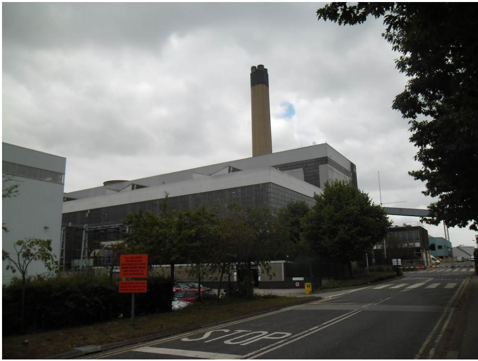
Photograph 31 | A view of the main turbine halls.
