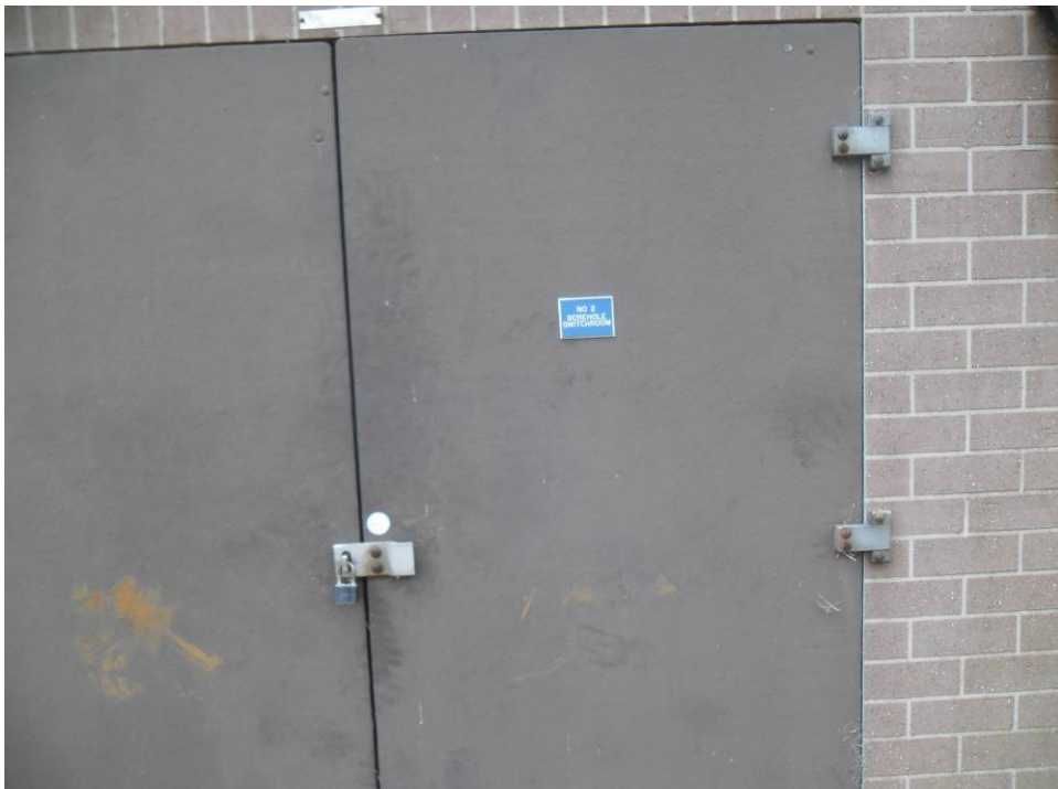
Photograph 36 | Abstraction borehole number 2 pump house.
