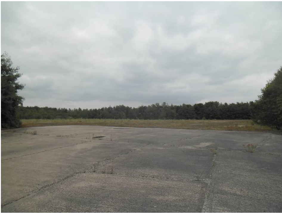
Photograph 23 | View of the strategic coal stockyard storage area.
