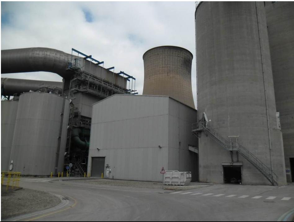
Photograph 15 Buildings associated with the Flue Gas Desulphurisation (FGD) plant.
