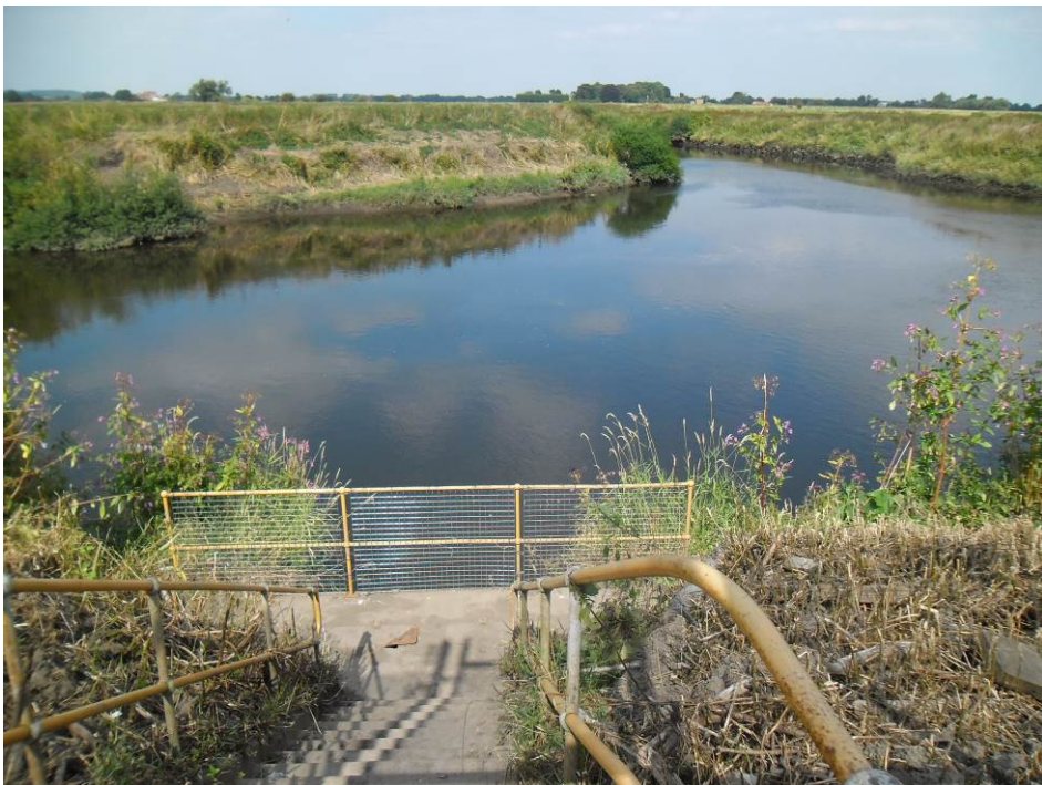
Photograph 40 | Effluent discharge location into the River Aire
