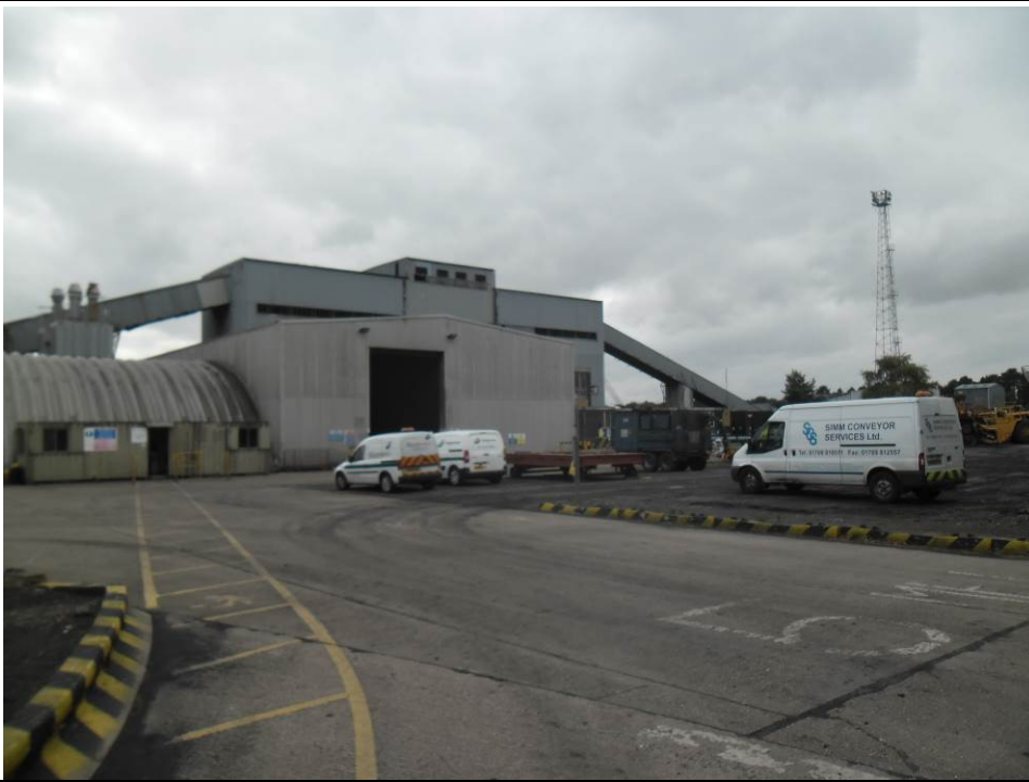
Photograph 3 | Warehouses in the coal stockyard area (looking east).
