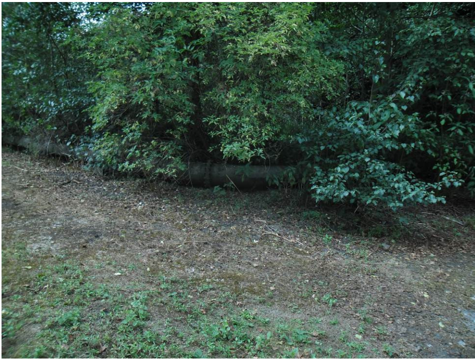
Photograph 27 | Redundant pipes previously used to transport materials to the former Lytag plant.
