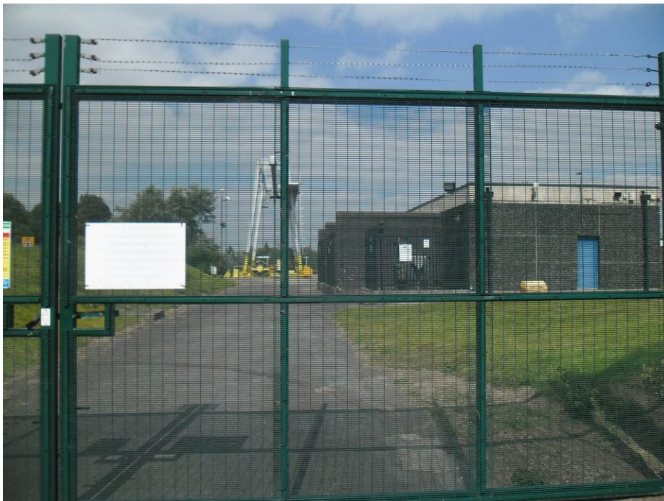
Photograph 38 | Surface water abstraction pump house.
