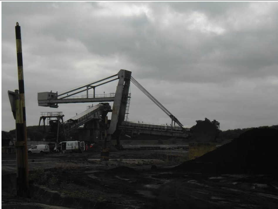
Photograph 6 | Large excavator in the coal stockyard area.
