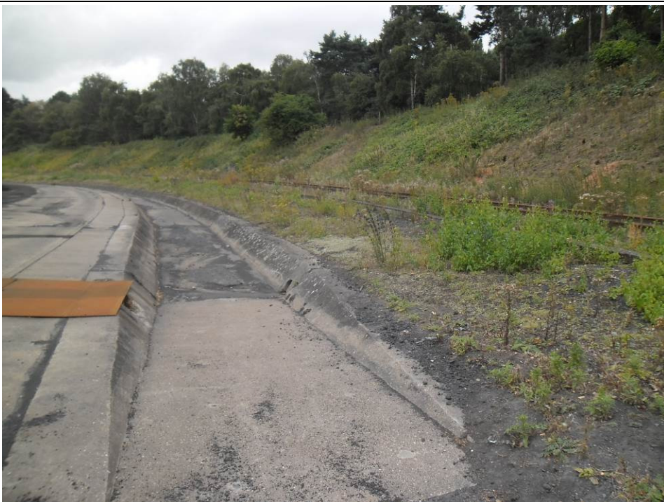
Photograph 4 | Drain which surrounds the coal stockyard area.
