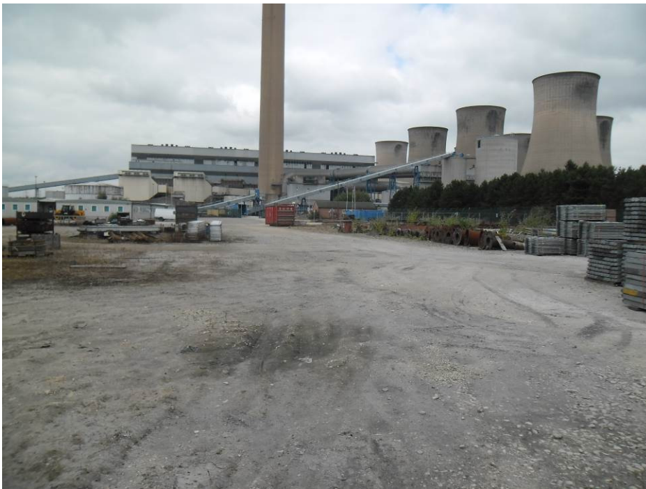
Photograph 14 | Laydown area to the north of the coal stockyard.
