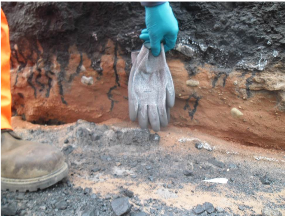
Photograph 12 | A photo showing the proximity of the base of the coal stockyard to the natural deposits.
