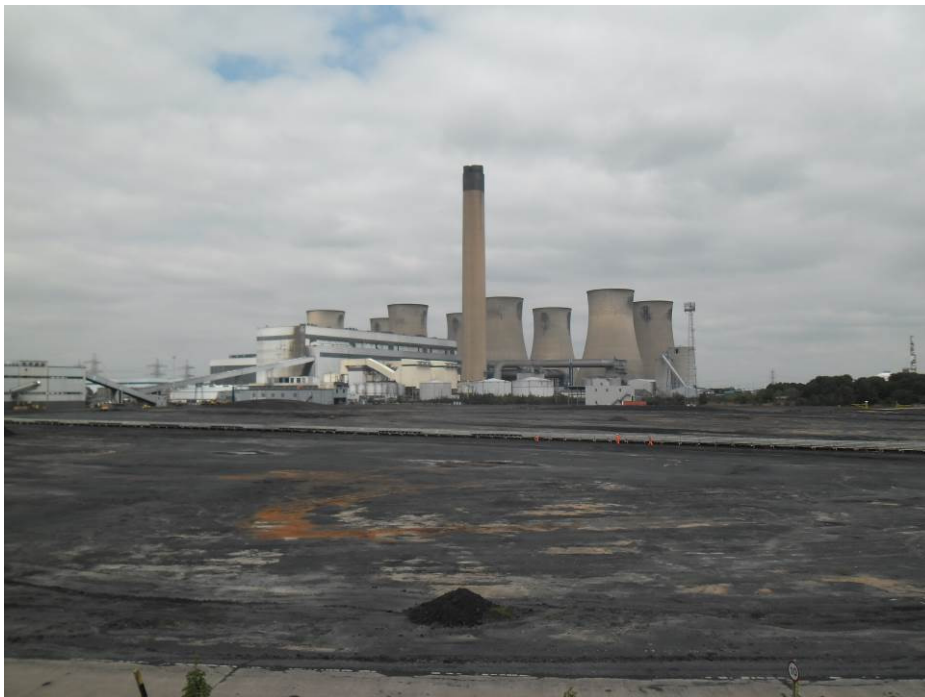
Photograph 30 | View of the coal stockyard in the foreground and the power plant in the back ground (looking north).
