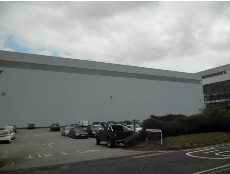
Photograph 32 | A view of the 400 KV substation building.
