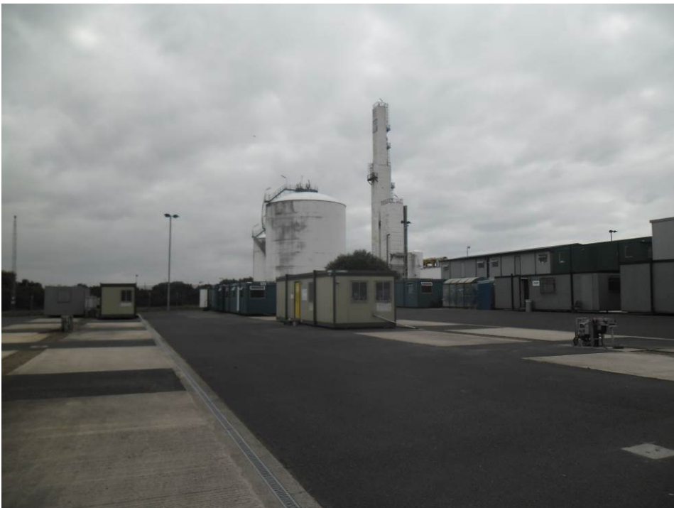
Photograph 18 | Mobile office storage air with the Air Liquide plant in the back ground.
