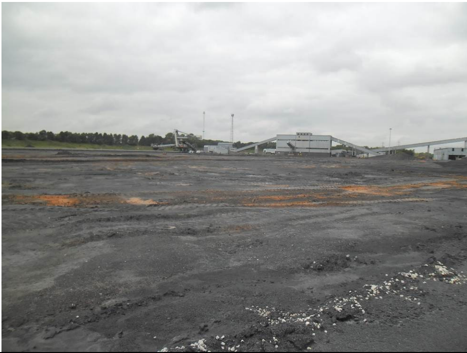
Photograph 13 | A photo showing the coal stockyard (looking south west).
