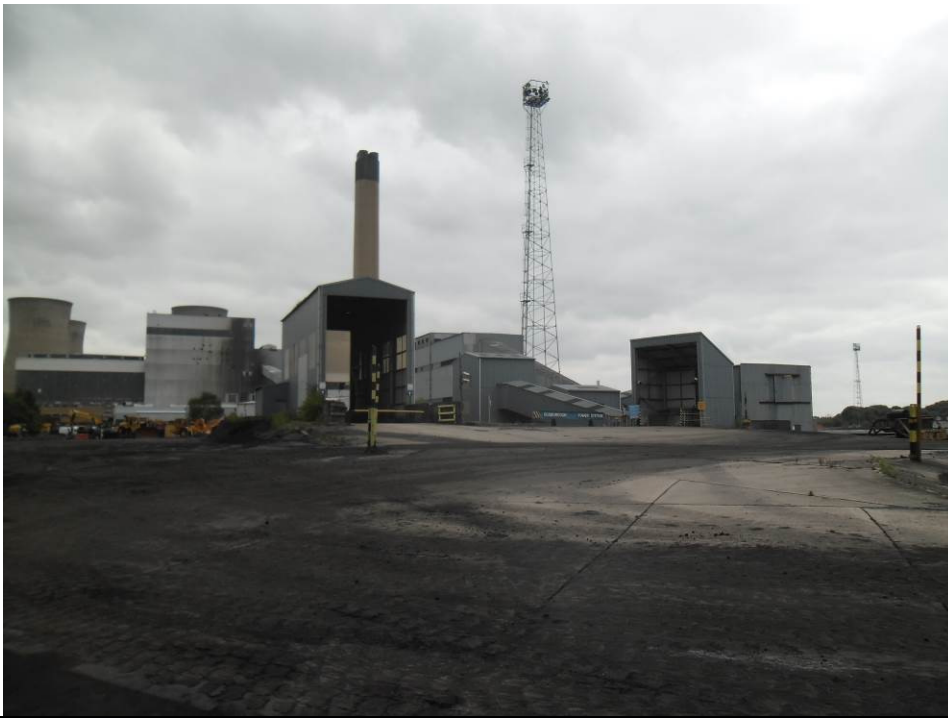
Photograph 5 | Warehouses within the coal stockyard area (looking north).
