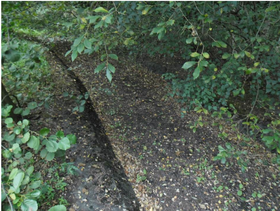
Photograph 24 | Concrete drain which surrounds the strategic coal stockyard area.
