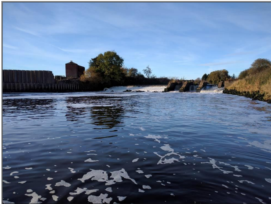
Figure 5 The weir structure on the River Aire separating the up and downstream sections.
