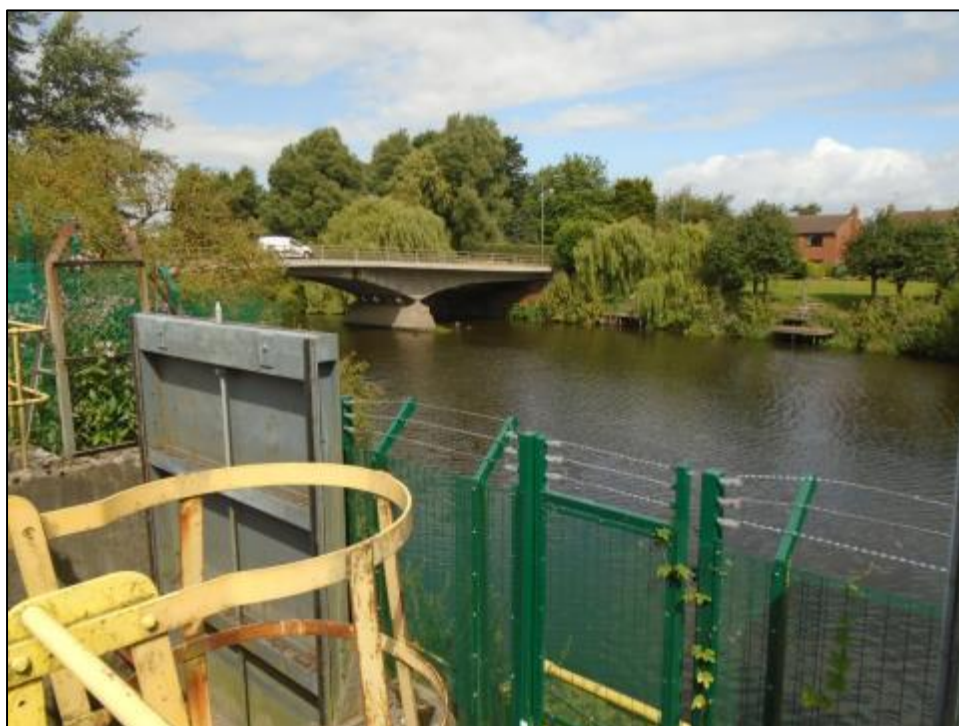
Photograph 5: River Aire at existing cooling water abstraction point
